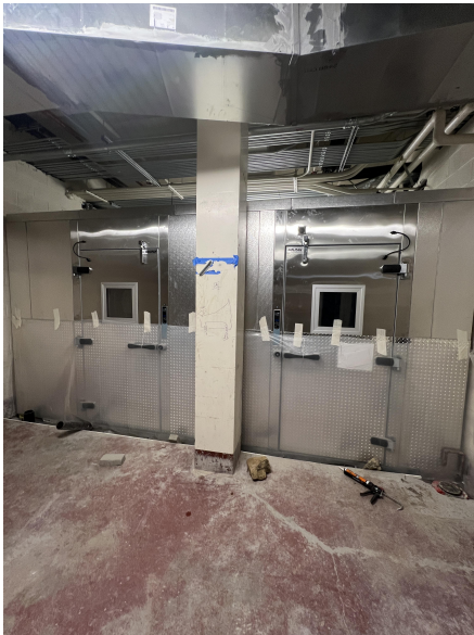
Cooler Freezer installation in the kitchen on level 1.
