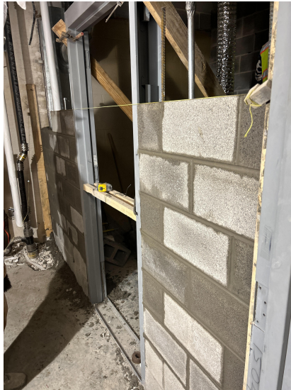
Setting door frame and CMU installation in kitchen on level 1.
